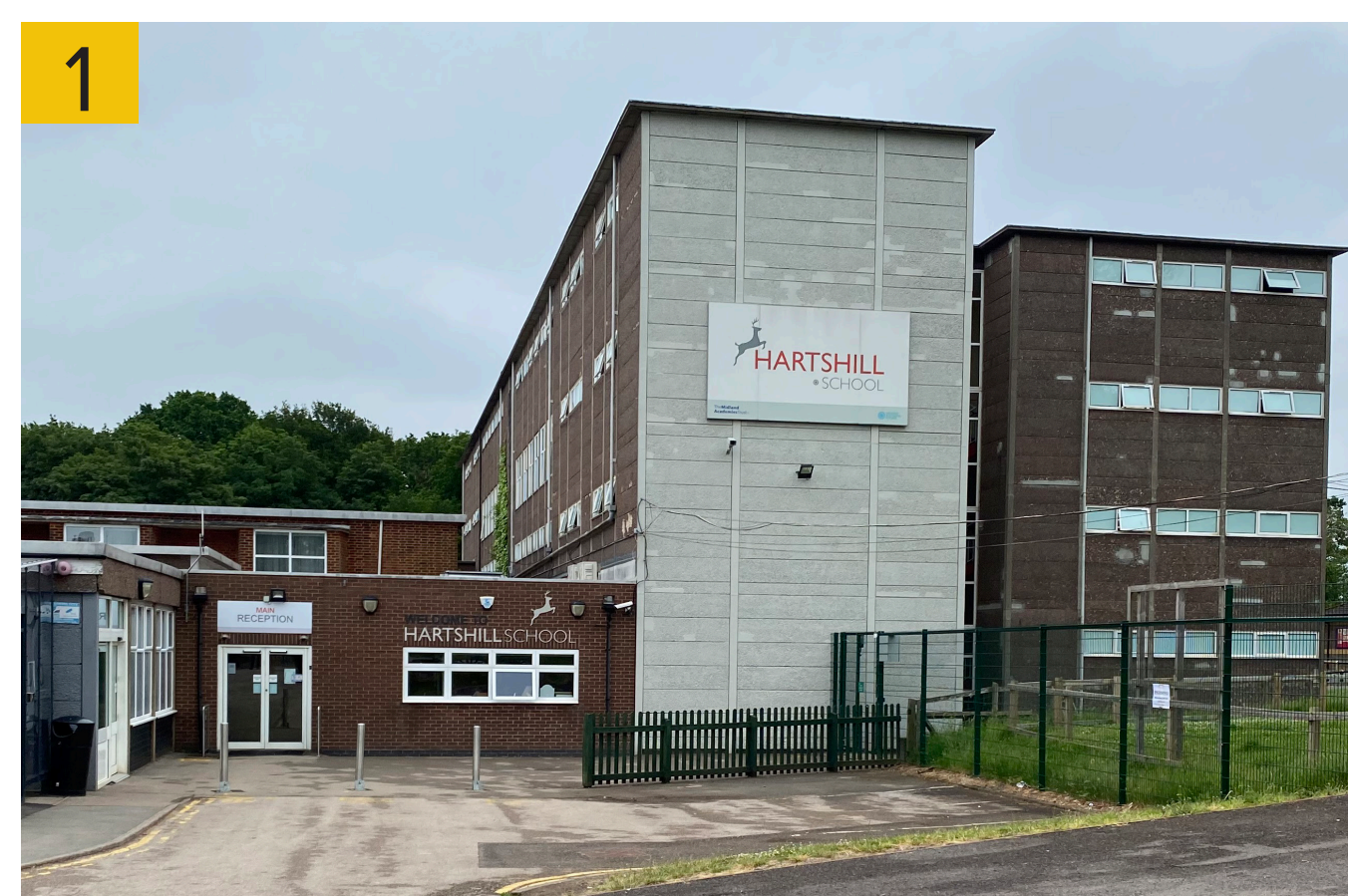
Existing main entrance
